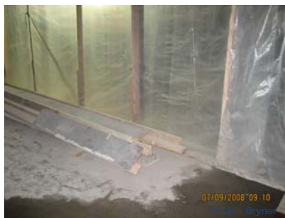
Figure 18: Photo showing the poly-wall used in the parking garage
