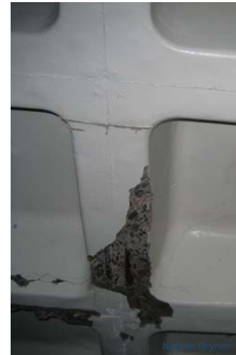
Figure 17: Section of the waffle slab that was contained spalling concrete with rebar exposure.
